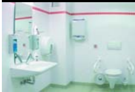
Barrier-free bathrooms Hospital patients often have to deal with temporary impairment of their mobility. To make everyday hospital life easier for them, the hospital features barrier-free sanitary facilities. The longer, ergonomically shaped levers such as those of the "Euroeco Special" safety mixer are particularly easy to use.
